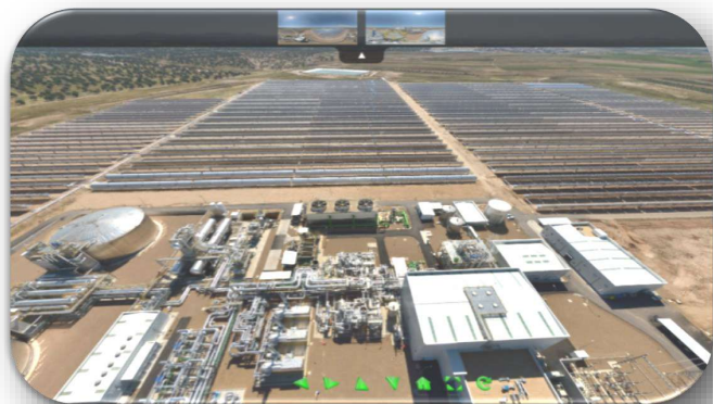
Project: CSP _ SOLAR THERMOELECTRIC 50 MW POWER PLANT Technology: CPC _ PARABOLIC TROUGH TECHNOLOGY Scope : Electric _ Electronic _ Communications _ Software Location: Spain
