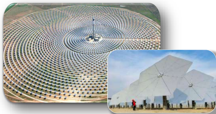
Project: CSP _ SOLAR THERMOELECTRIC 50 MW POWER PLANT Technology: STELLIO _ HELIOSTAT TECHNOLOGY Scope: Electric _ Electronic _ Communications _ Software. Location: China
