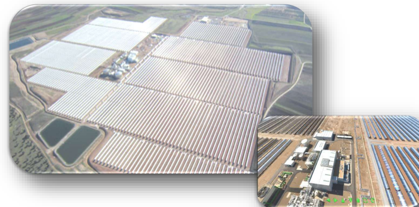
Project: CSP _ SOLAR THERMOELECTRIC 50 MW POWER PLANT Technology: CPC _ PARABOLIC TROUGH TECHNOLOGY Scope : Electric _ Electronic _ Communications _ Software Location: Spain
